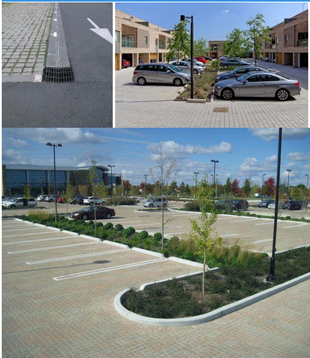
Plate 4: Typical Permeable Paving Arrangements
